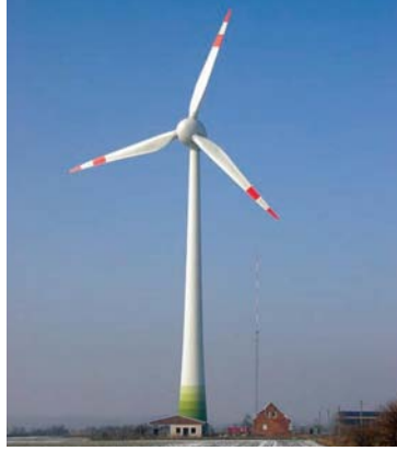
Fig. 13. Largest wind turbine (currently): Enercon E-112 with a rotor diameter of 112 m and a nominal power of 4.5 MW.
